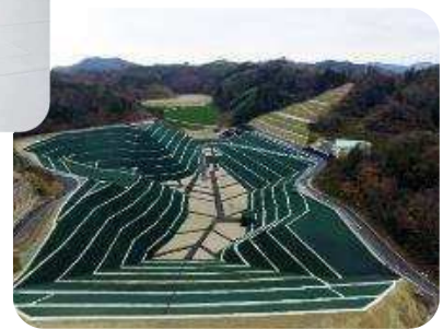
Seepage control system for final disposal site
