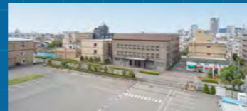
Kobe Plant R&D Center
