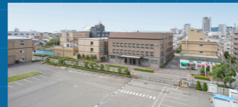
Kobe Plant R&D center
